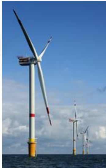
Image 1: The natural resource of wind powers these 5MW wind turbines on this wind farm in Belgium.
